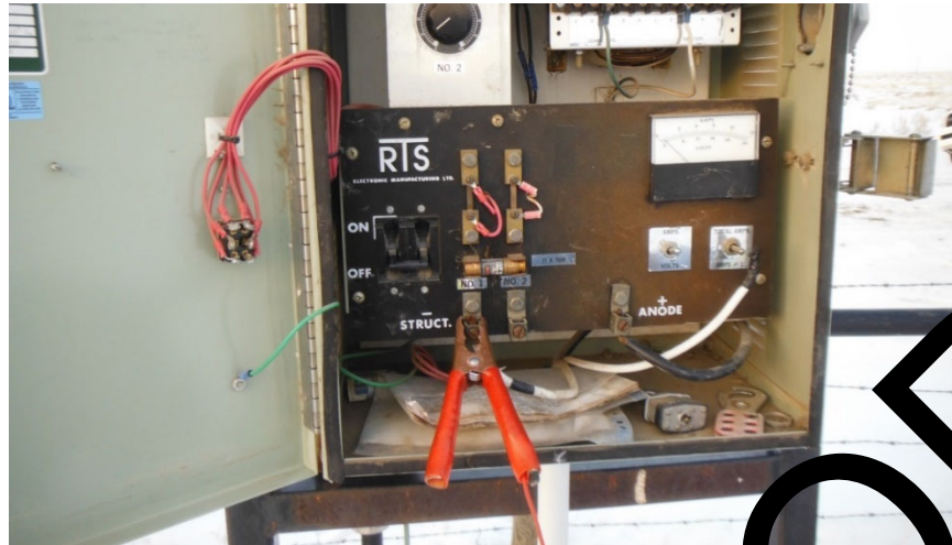
2-23 Direct hook-up to a structure cable (negative feeder cable)
