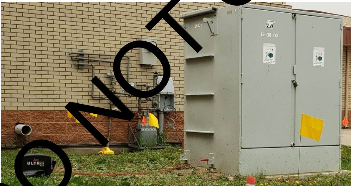
2-20 Direct connection to a transformer
