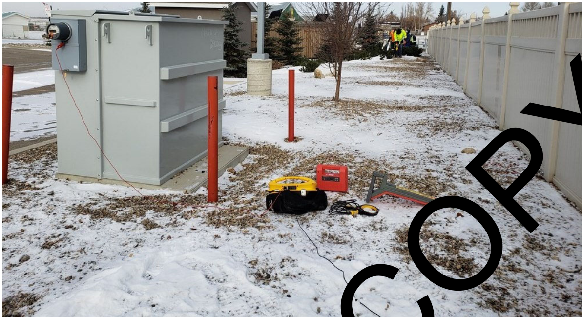
2-19 Direct connection to the meter and transformer
